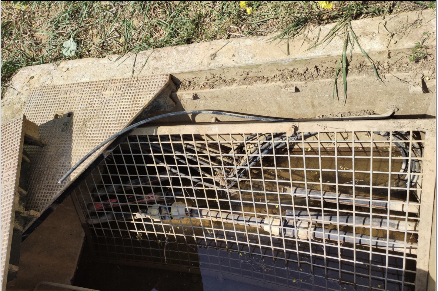
Figure 6: Damaged submarine cables in manhole near Marseille landing station (Source: Social Media )
